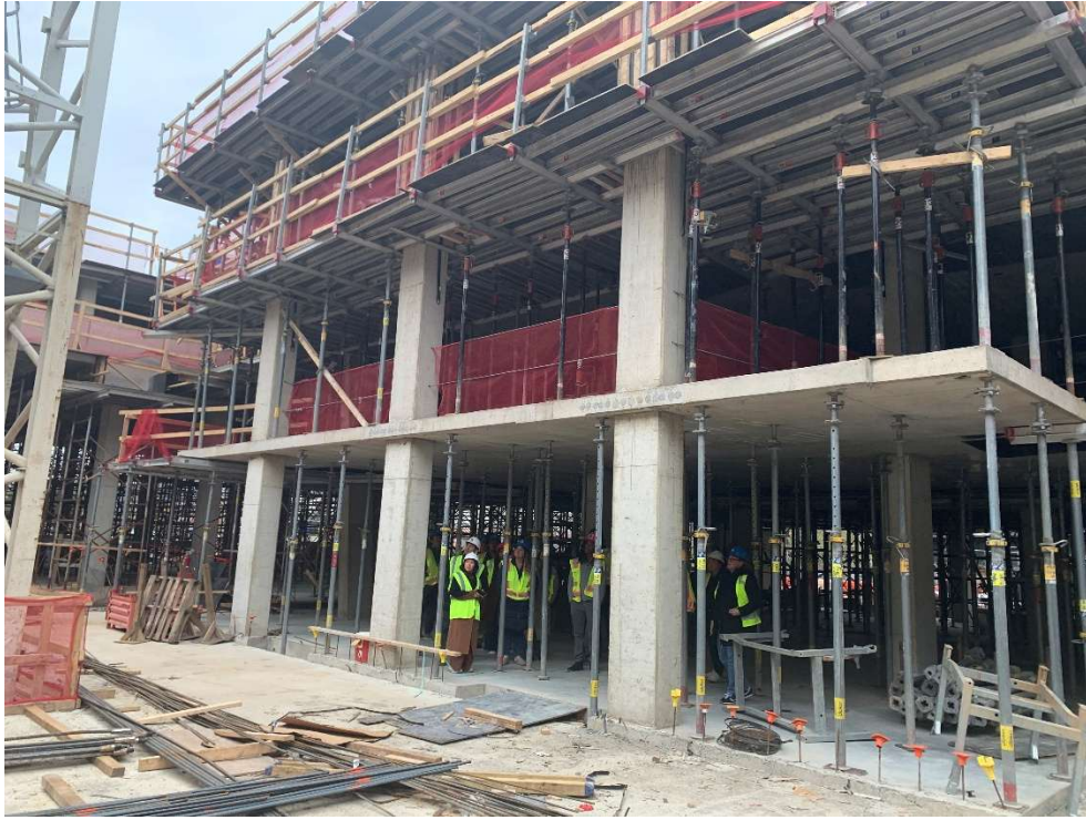
Framing of Level 5 Slab & Pool Structural Box (Pour #29) (below) – November 18 th , 2025
