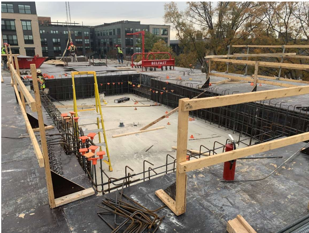
Framing of Level 5 Slab & Pool Structural Box (Pour #29) (below) – November 18 th , 2025
